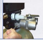
Attach drain line hose barb and compression nut of the brine tank by turning clockwise to tighten until snug. To prevent leaks, wrap threads of hose barb and compression nut with Teflon® tape clockwise, approximately 3 times around.
